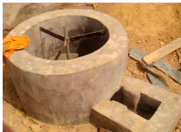
Biogas in Gulariya during the construction.
