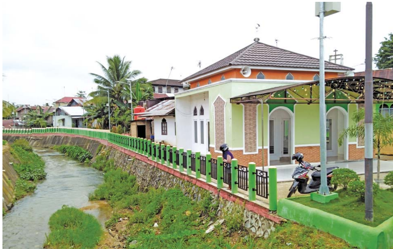
Kemuning River after the normalization project.
